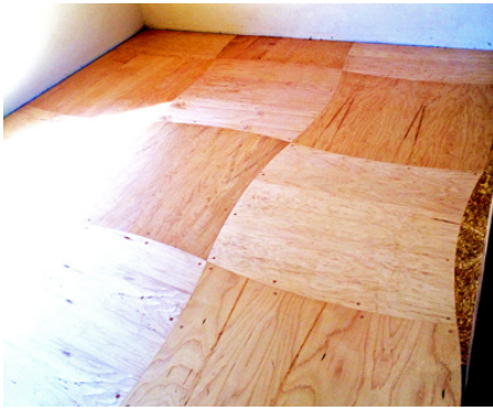
The tiles for this floor were approximately 30 inches x 30 inches, fabricated with curved edges.
